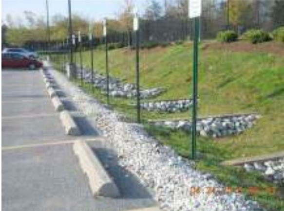
Fig. 5. Cuneta Verde. Fuente: Stormwater Maintenance and Consulting, LLC.
