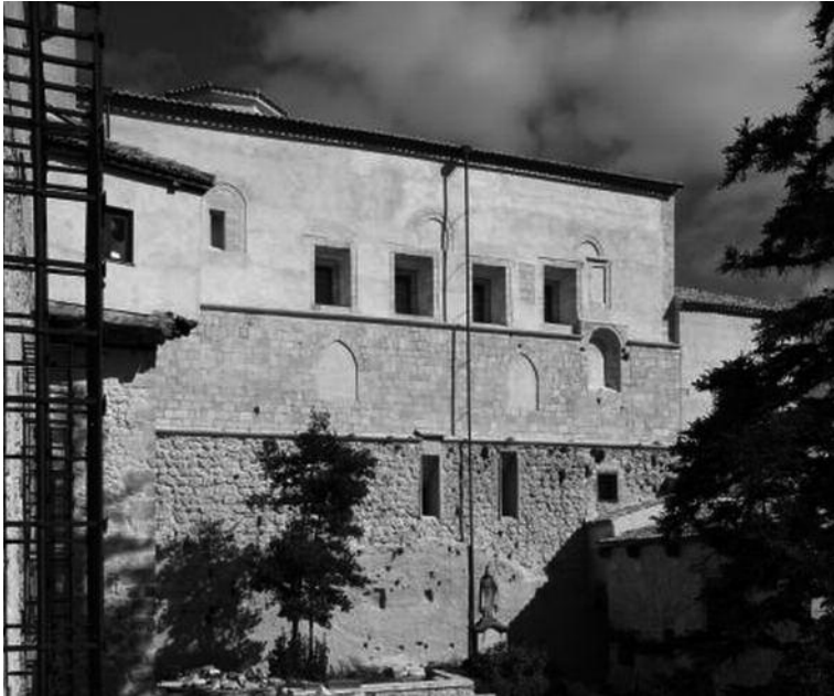
Fig. 2. Exterior wall after its restoration. Photograph by Jose Latova.
